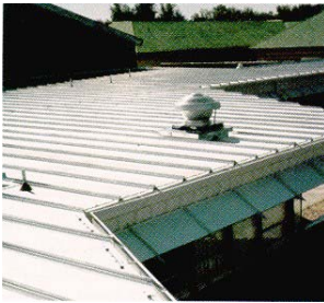
Bare standing seam roof
